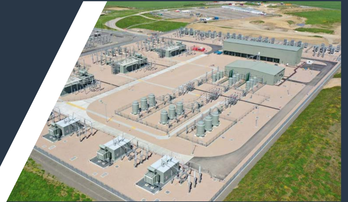
MORAY EAST ON-SHORE SUBSTATION
