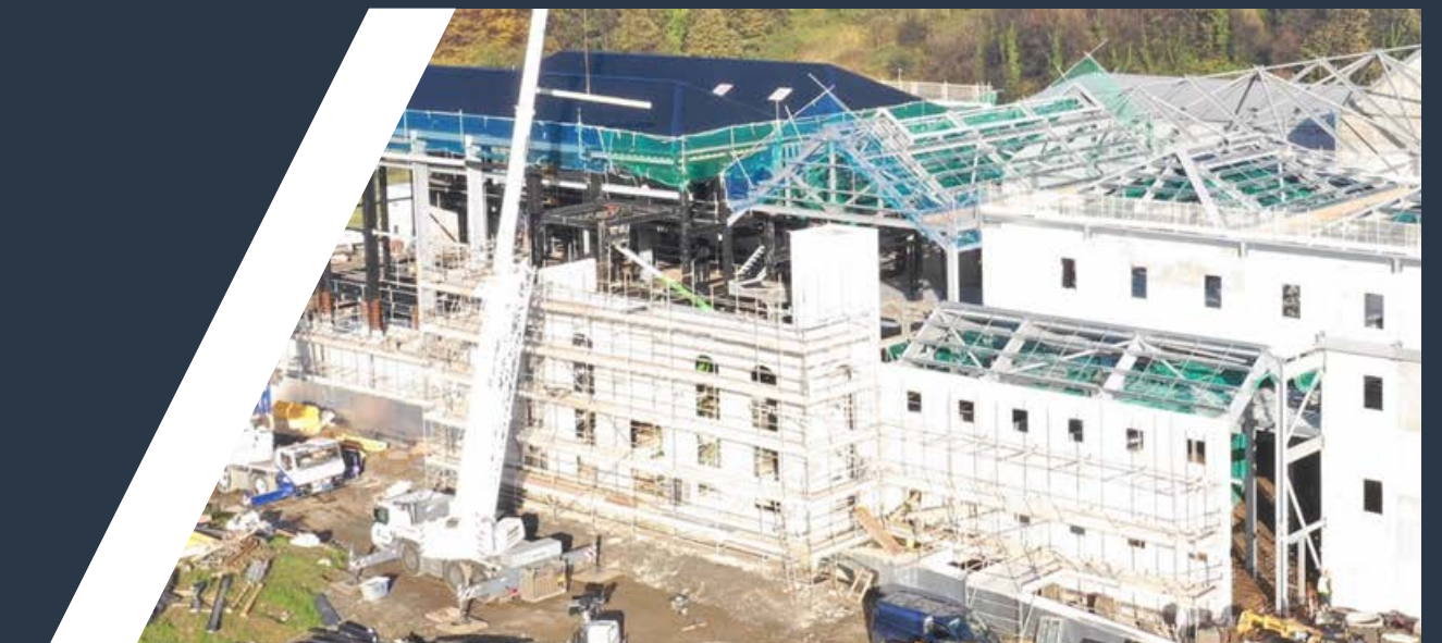
BUSHMILLS DISTILLERY EXPANSION
